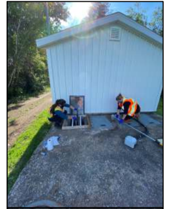
Collecting wastewater samples from the sewer system
